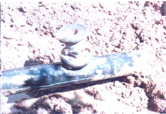
Point after excavation.
